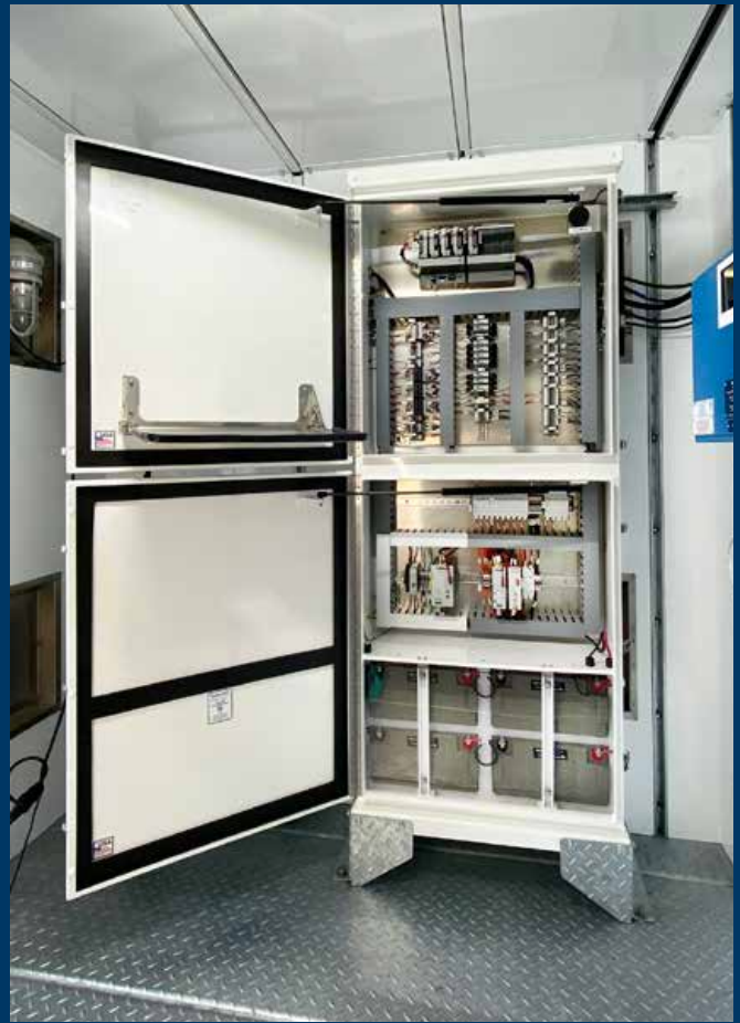
customer equipment and lighting. | Bottom left: Fully integrated Hybrid AC/DC UPS system with PLC's, communications, and I/O's panels. Bottom right: Hybrid AC/DC UPS power system for block valve.
