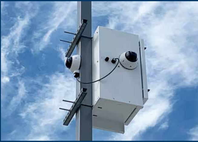
Top left: Outdoor multi-camera custom enclosure with battery-backup power and communications. | Top right: Solarcraft integrated electrical equipment shelter with dual-door RTU/PLC UPS system, junction box, ➔
